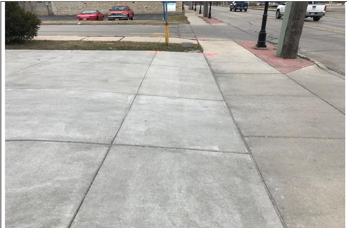
LOOKING NORTHEAST AT THE TLE AREA
