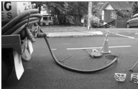
Fig.7 Sediment is removed from the sump with a vector hose. Man entry is not required for this step.
