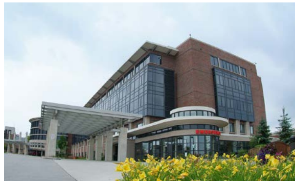
Waukesha Memorial Hospital
