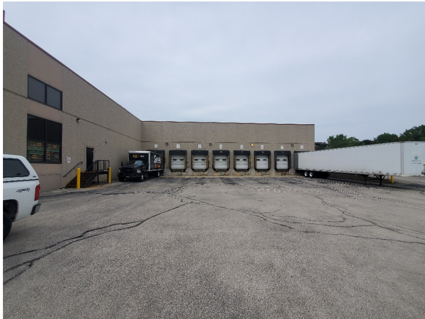
Figure 3: SE Side of Site, Looking N (07-2021)
