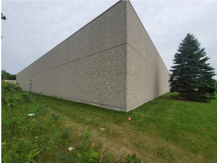
Figure 6: W Side of Site, Looking NE (07-2021)
