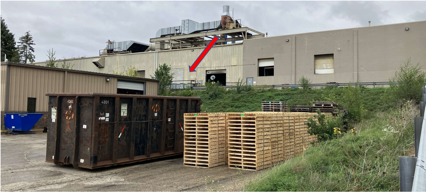
View from lower parking lot, facing east, Sentry Dr behind. Proposed location marked.
