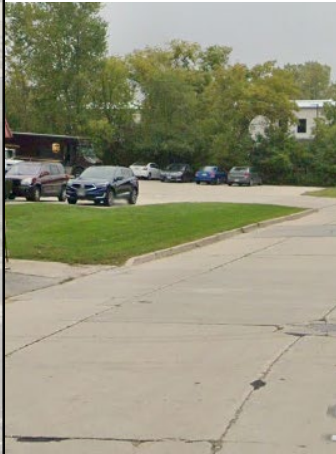
Figure 15-16: Examples of missing pedestrian infrastructure in Aldermanic District 3
