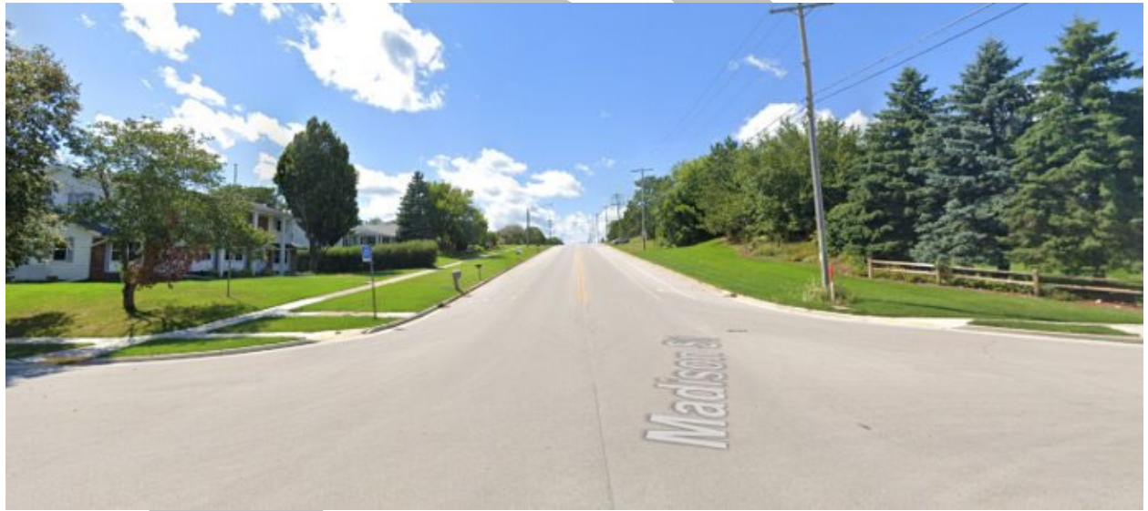
Figures 54-55: Examples of missing pedestrian infrastructure in Aldermanic District 14
