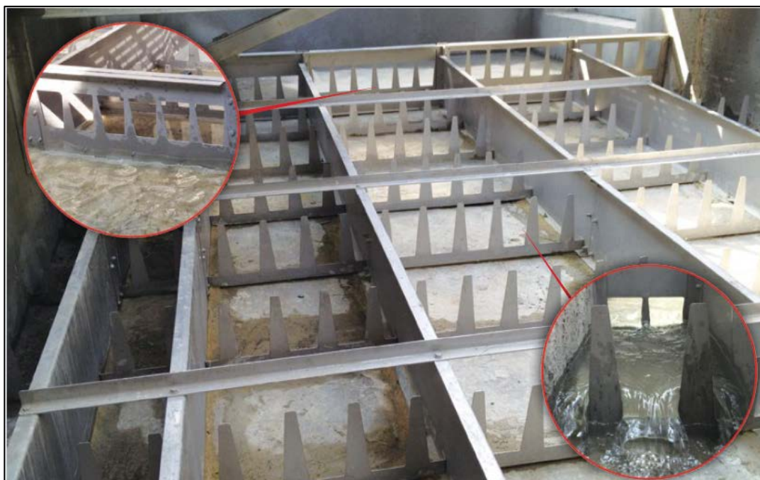
Figure 9. JMS Low Profile Cascade Aerator (photo courtesy of JMS)
