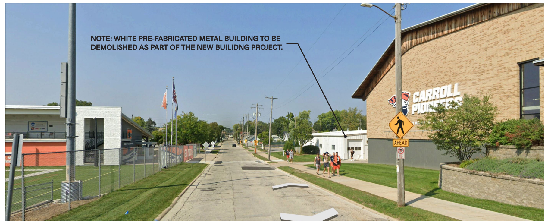
SITE VIEW - LOOKING NORTH
