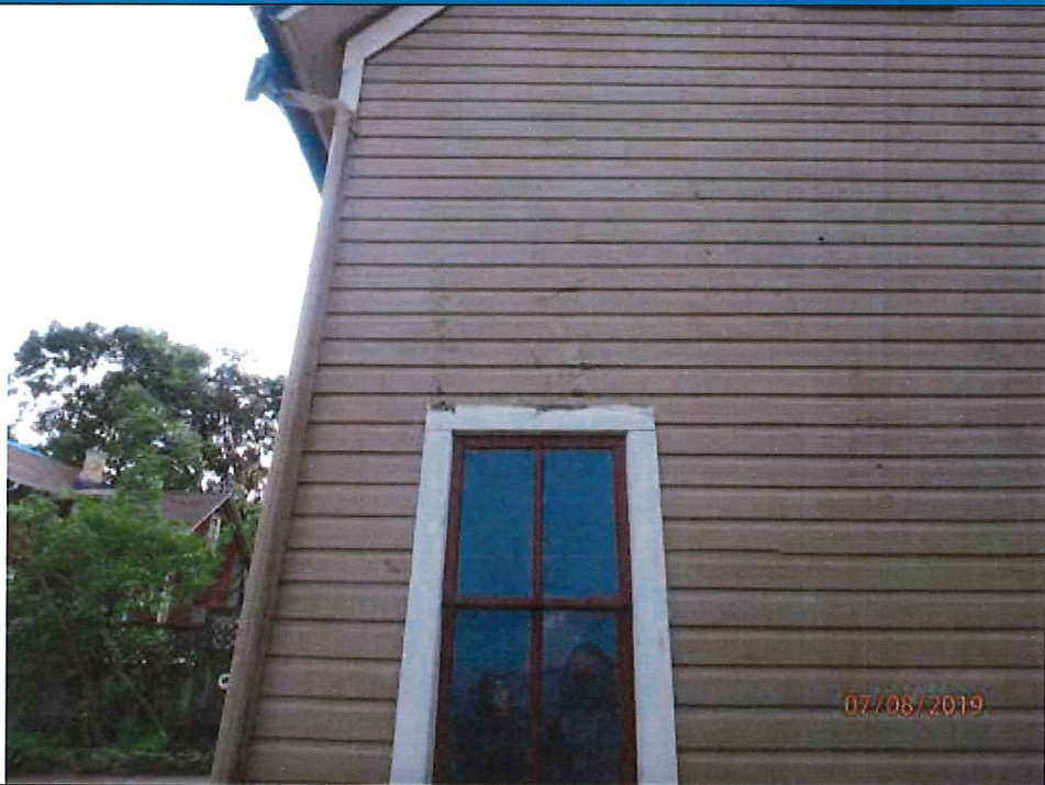
Photo 10: Scrapes, chips and abrasions.
