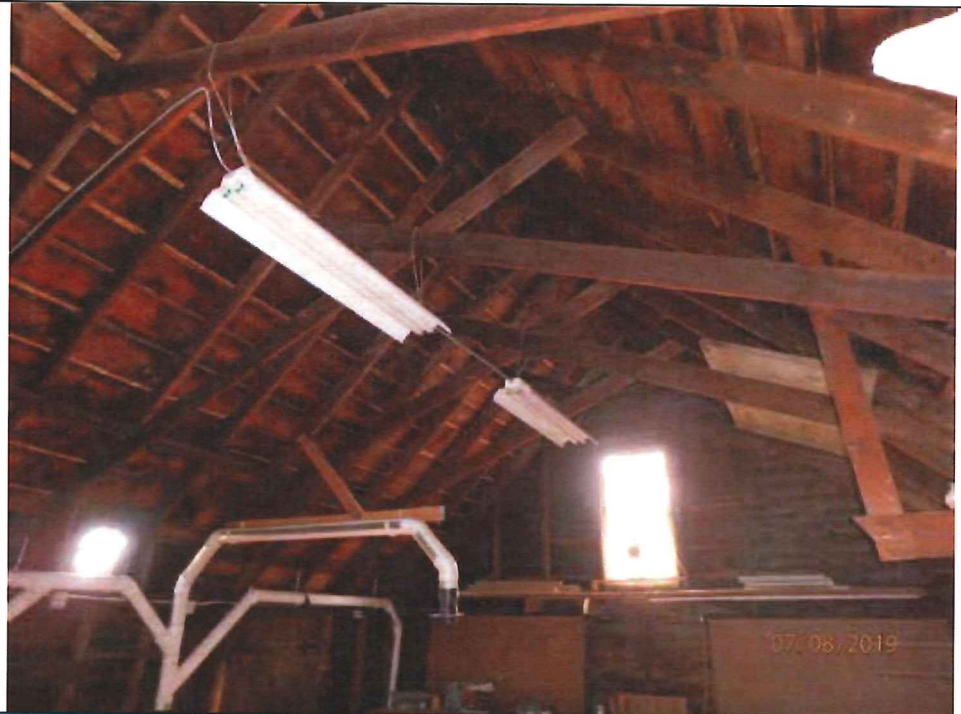
Photo 19: Overview of the roof framing.
