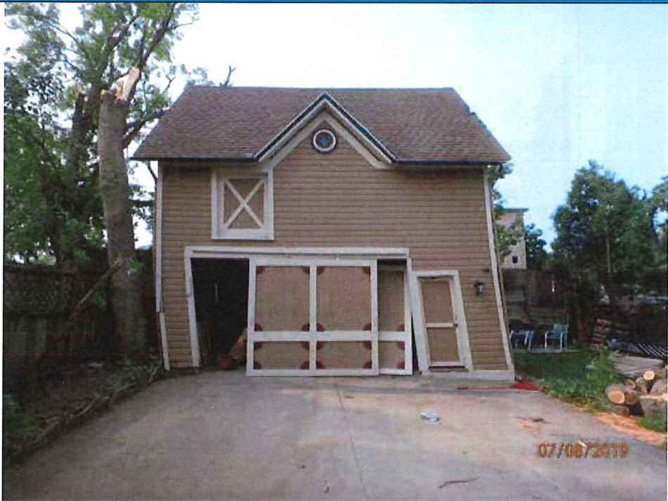
Photo 2: North elevation of the subject garage.
