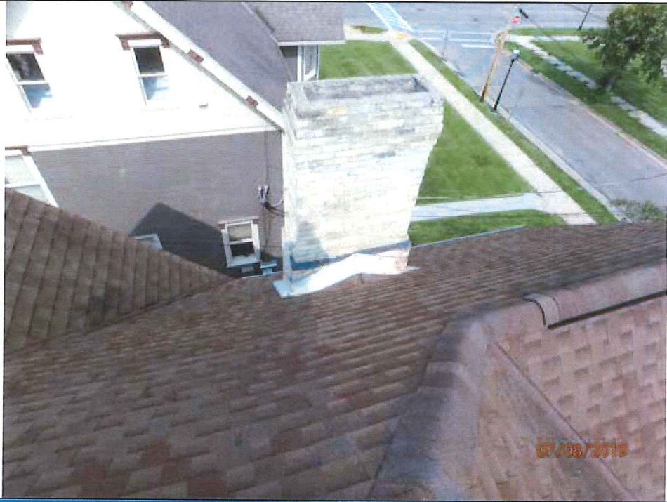
Photo 25: Chimney overview from roof.
