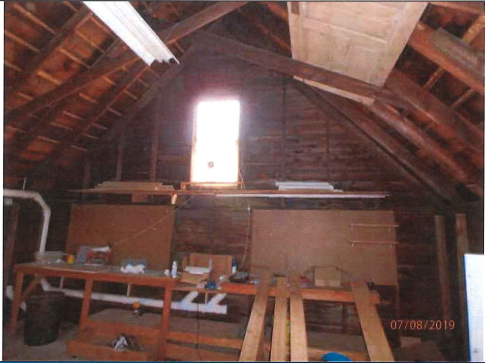
Photo 21: End wall framing.
