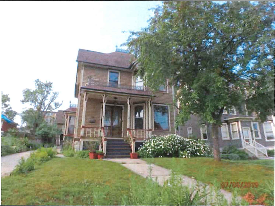
Photo 1: Site identification, front (north) elevation of dwelling associated with the subject garage.
