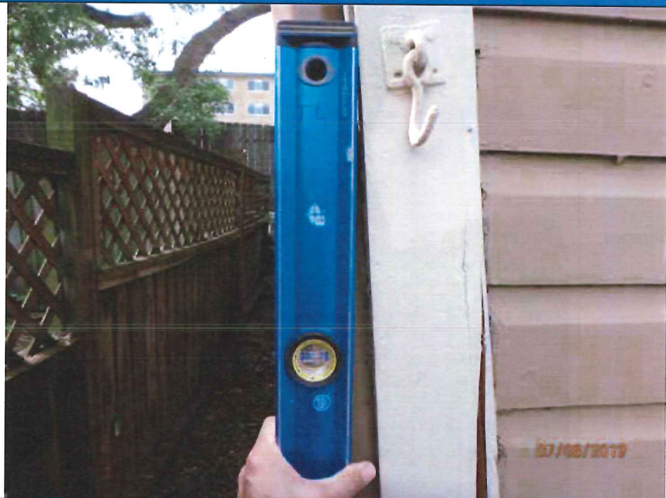
Photo 12: Plumb measurement location.
