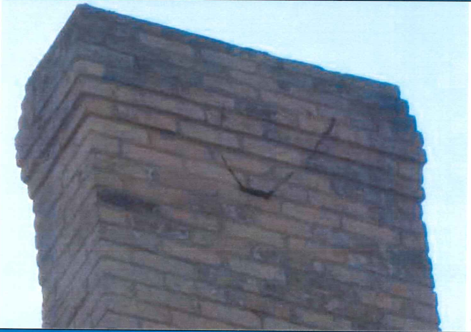
Photo 26: Misplaced sealant.
