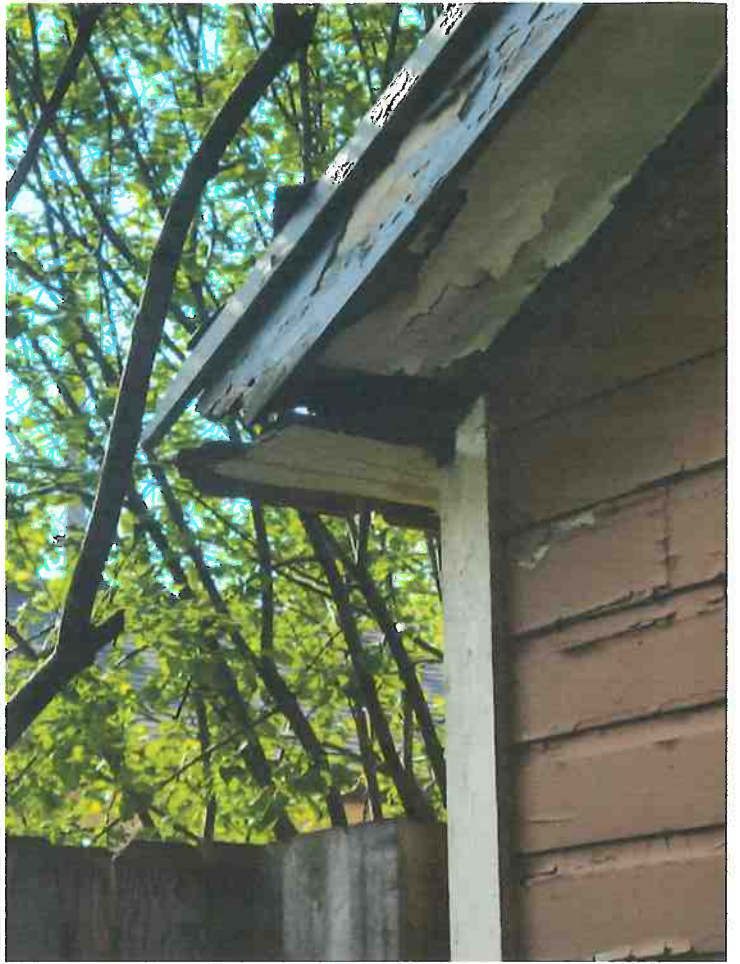
Rotted Fascia & Soffit
