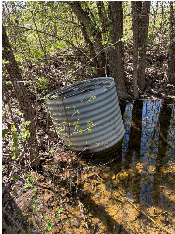
Photo 4: Culvert Pipe located on the south end of W-2; connecting to W-3
