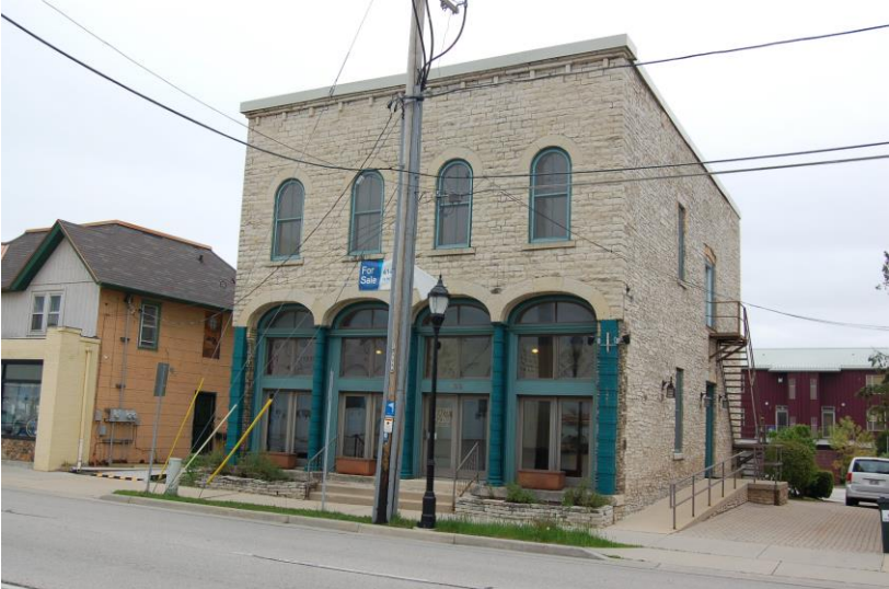
Front Of Building – 2
