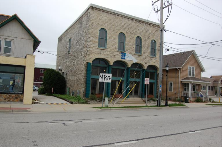
Front Of Building – 1
