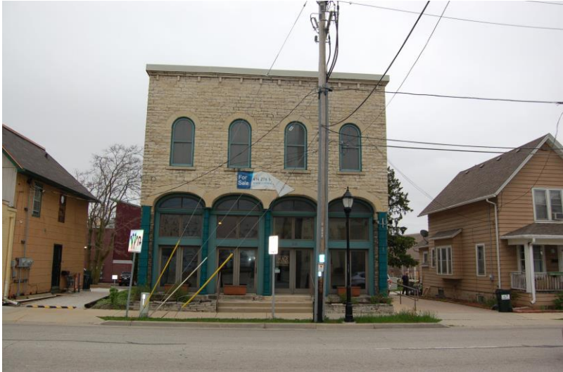
Front of Building -- 3
