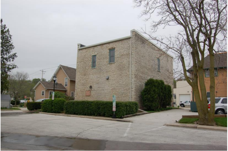
Back Of Building – 2
