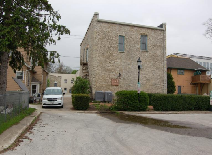
Back Of Building – 1
