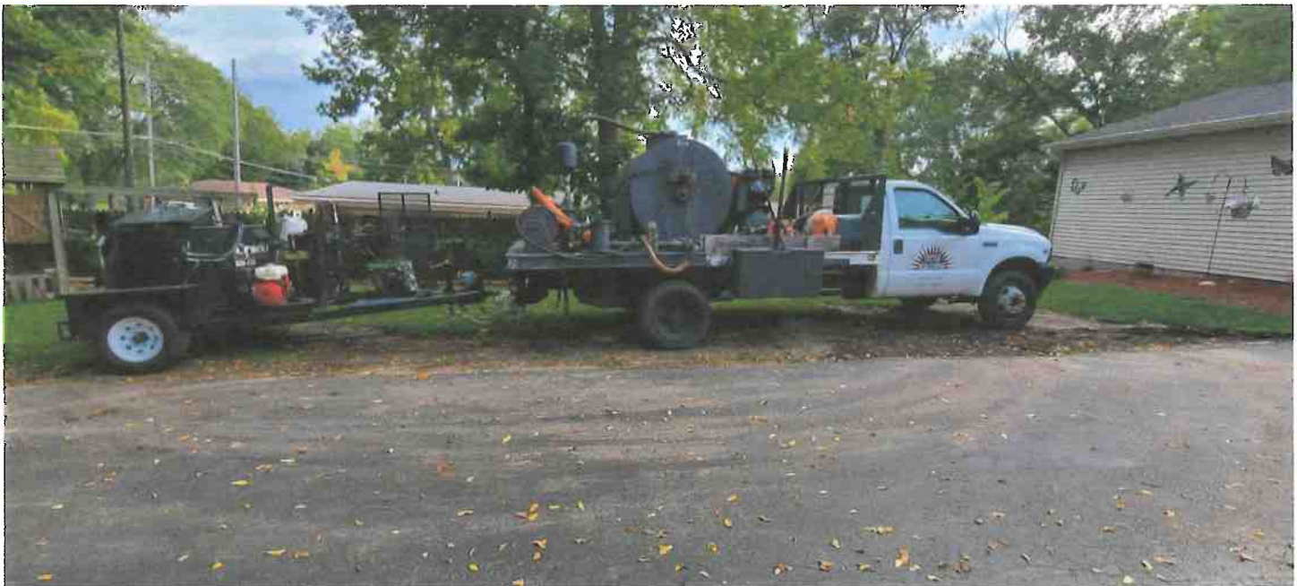
OUR SEALING TRUCK WITH TAR MACHINE ATTACHED
