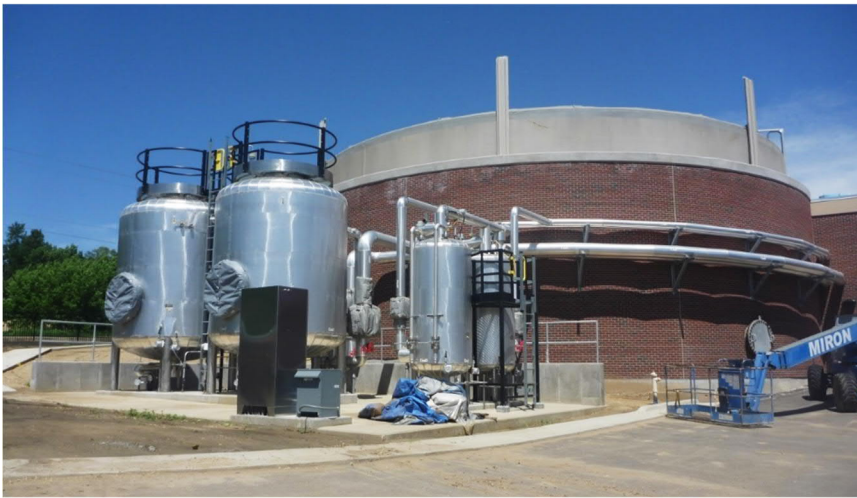
Dubuque biogas conditioning equipment for hydrogen sulfide and siloxane removal.
