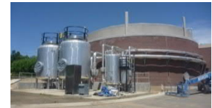
Dubuque anaerobic digesters and biogas conditioning.
