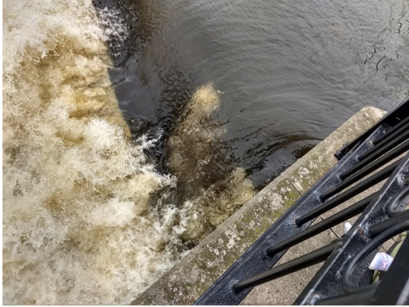
Saratoga Mill Dam 0063010031808.jpg Left Abutment
