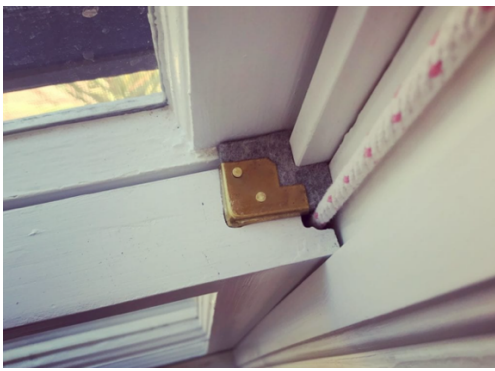
Example of stop gap weather stripping.
