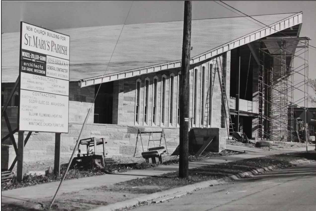
FIGURE #2: St. Mary's Catholic Church under construction, 1964.
