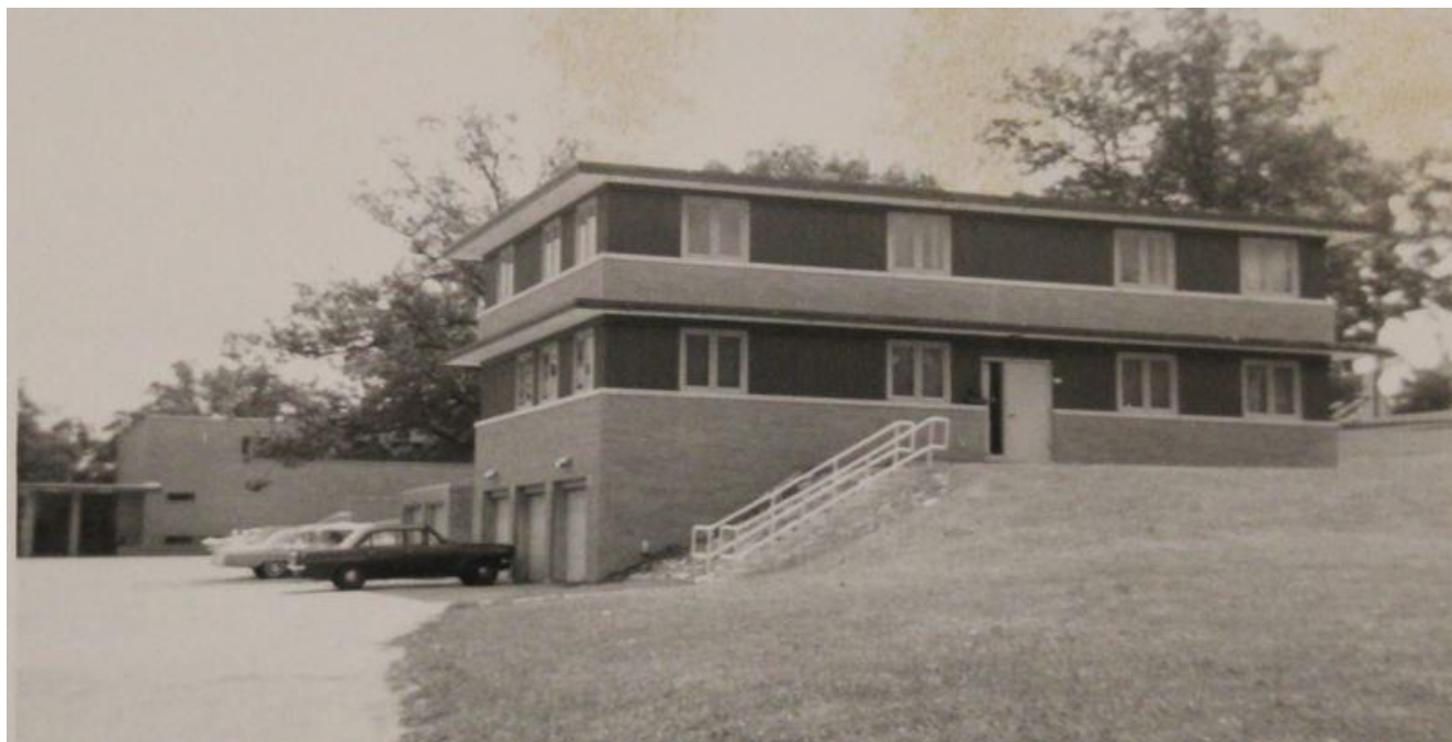
FIGURE #5: 1963 photo of the west and north elevations of the rectory with flat roof and original casement windows still intact. The gymnasium wing is visible to the rear, while a free-standing two-car garage (no longer extant) is located immediately adjacent to the rectory.
