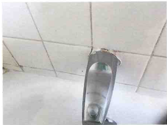
Second floor bathroom tub stopper body corroded through
