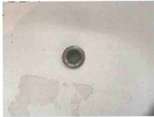
Second floor bathroom tub stopper body corroded through
