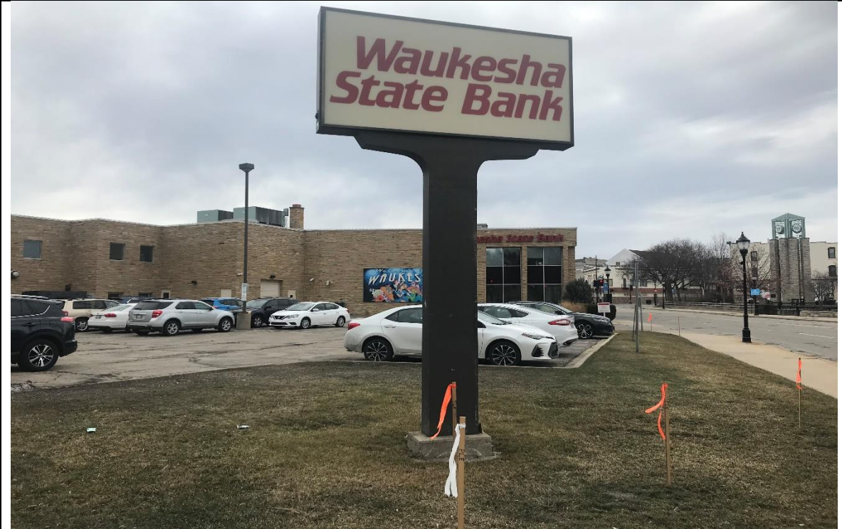
PLE AND FEE LOOKING SOUTHEAST – SIGN TO REMAIN IN PLACE
