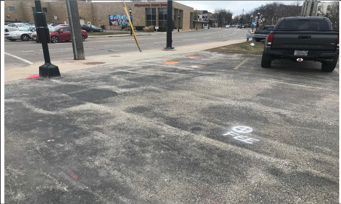
TLE AND FEE FROM W. ST. PAUL AVENUE LOOKING AT MADISON STREET
