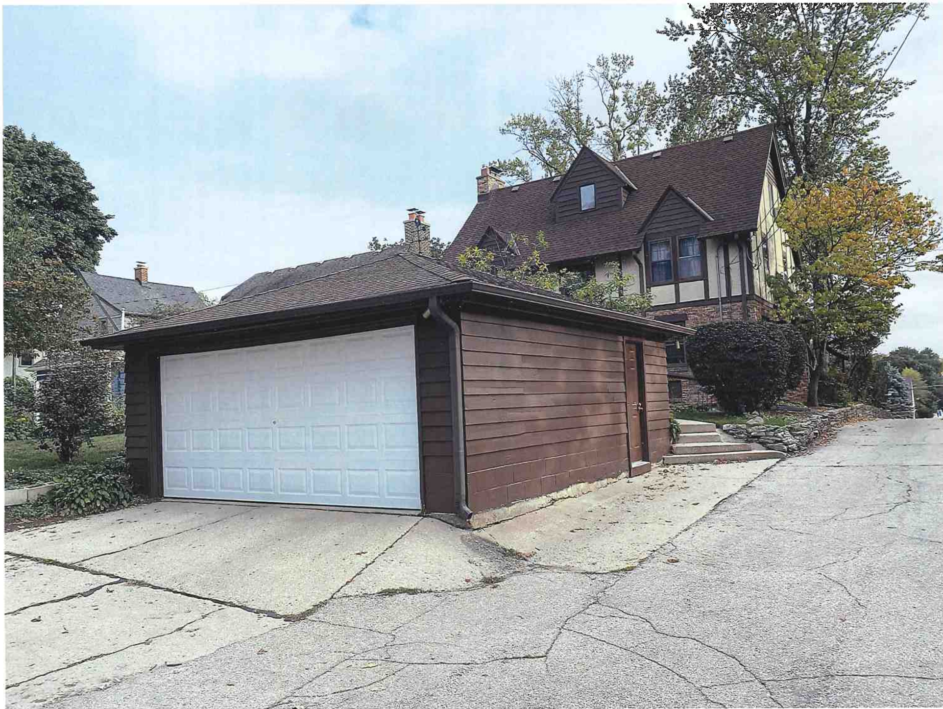
EXISTING BACK (NORTH)
