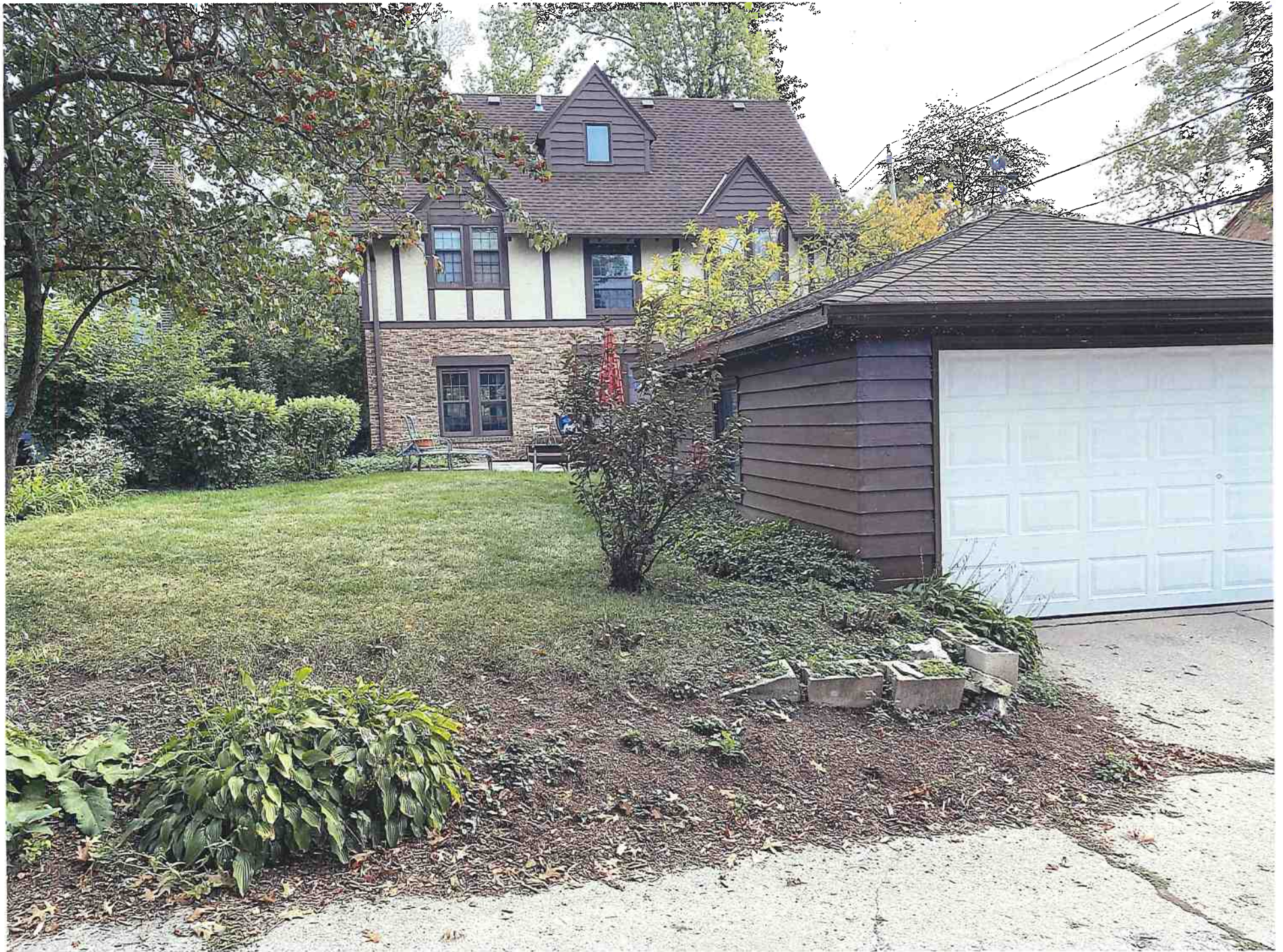
EXISTING BACK (NORTH)
