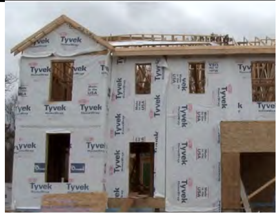
Home under construction in Waukesha
