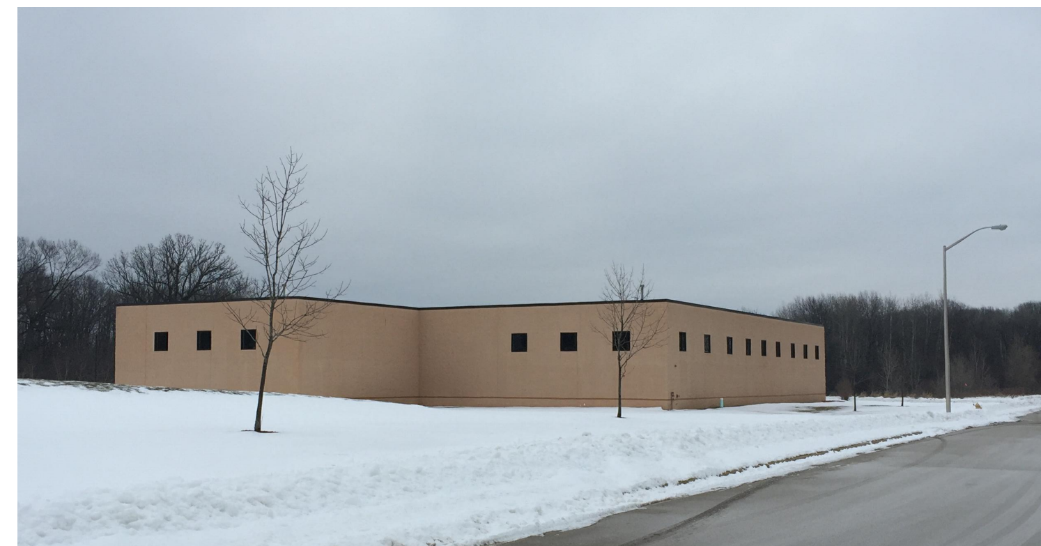
Existing View from SW Corner of Site SCALE: N.A.
