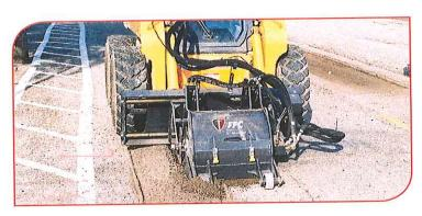
The FFC Cold Planer, by Paladin, can be used to make full depth utility cuts, mill frost heaves around manholes, restore proper drainage to pavement, add texture to pavement for skid resistance, and much more.
