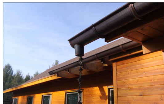
A detail view of the rainwater harvesting system.
