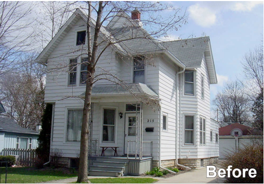
Maintain character defining features such as cornerboards and window trim
