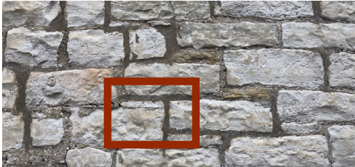
Replacement mortar should match color, texture and joint style of existing mortar.
