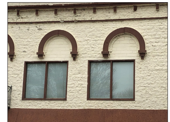
Replacement windows that do not match the original size and style can damage your building's historic integrity.
