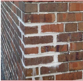
Mortar that does not match existing can damage historic character and surrounding masonry. (Photo Credit: Wisconsin Historical Society)
