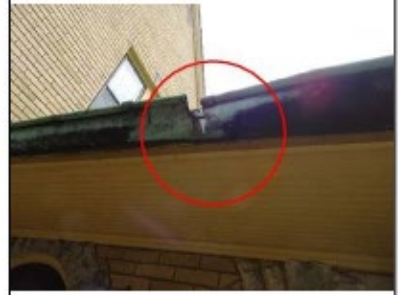
Damaged gutter
