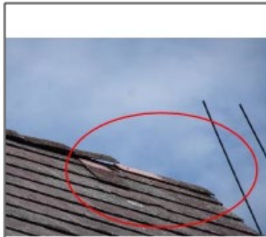
Missing roof tiles
