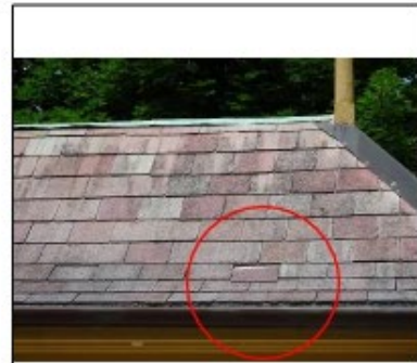
Loose/broken roof tile
