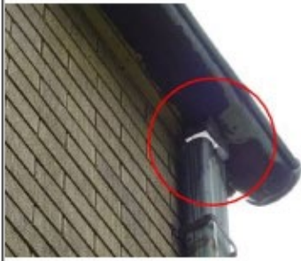
Improperly connected downspout
