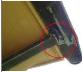
Improperly connected downspout
