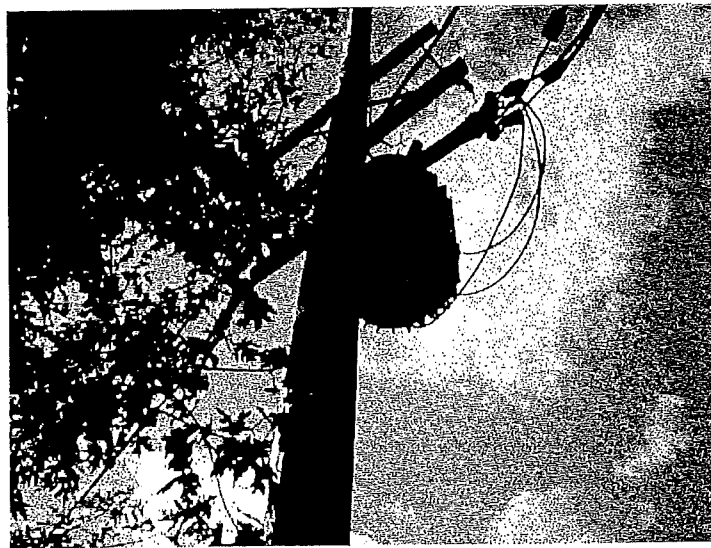
8. Photo of the transformer observed near the eastern property boundary, along Fox River.
