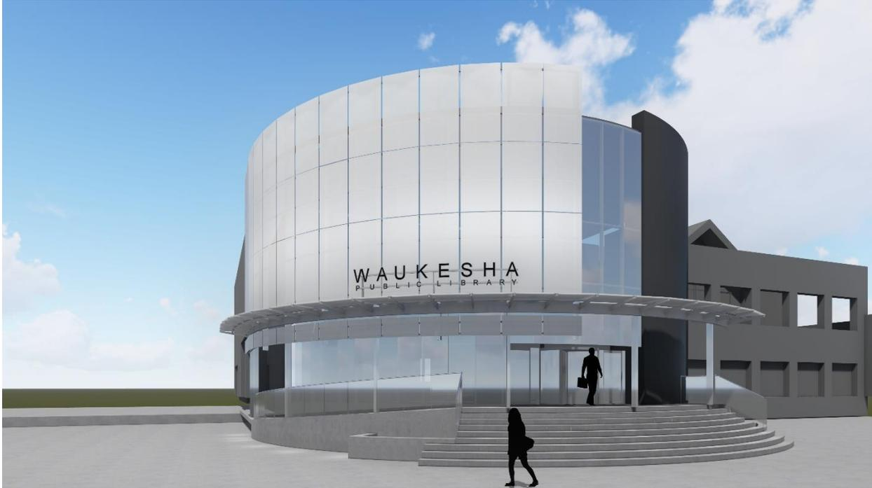
1. Note that the lines of the vertical panels do not match the lines of the windows behind them. This reduces the amount of extra steel support needed and saves the library **\$32,375**.
