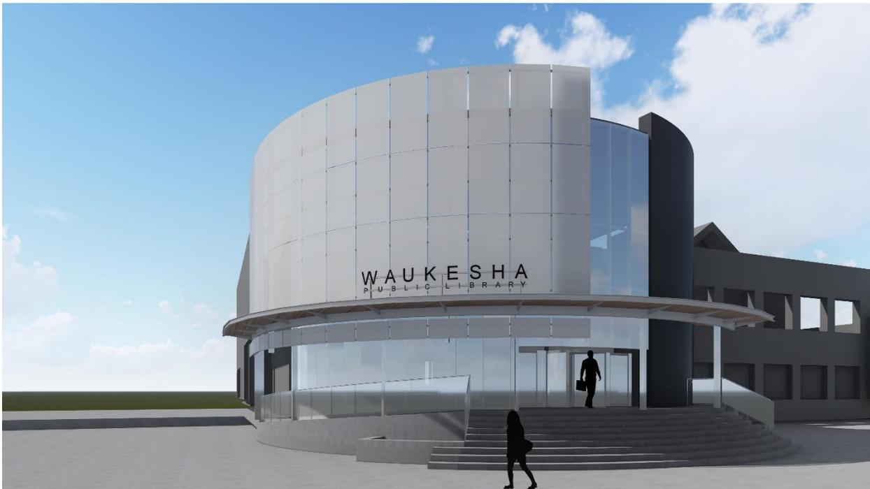
2. This image replaces the horizontal resin panels with a solid canopy, more like a traditional roof. Lights are included shining down from the canopy. This option reduces the cost by **\$64,474**. It also makes lighting the library sign simpler.
