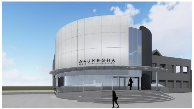
1. Note that the lines of the vertical panels do not match the lines of the windows behind them. This reduces the amount of extra steel support needed and saves the library \$32,375.
