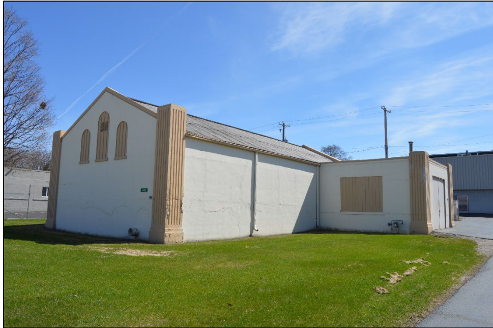
Newhall Avenue Pump House and Reservoir, 445 W. Newhall Avenue (AHI 29361).
