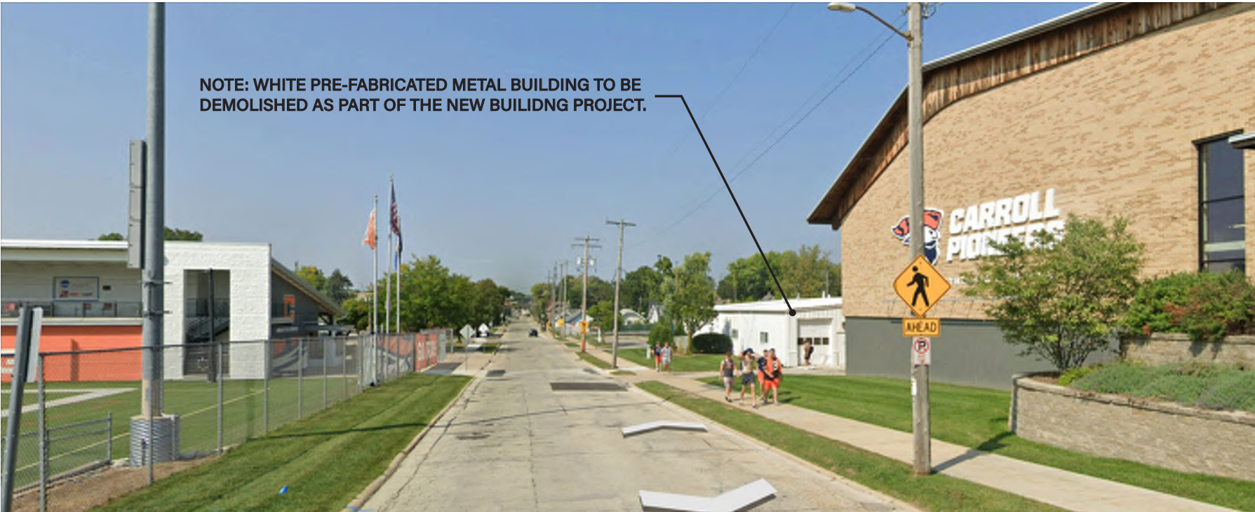
SITE VIEW - LOOKING NORTH
