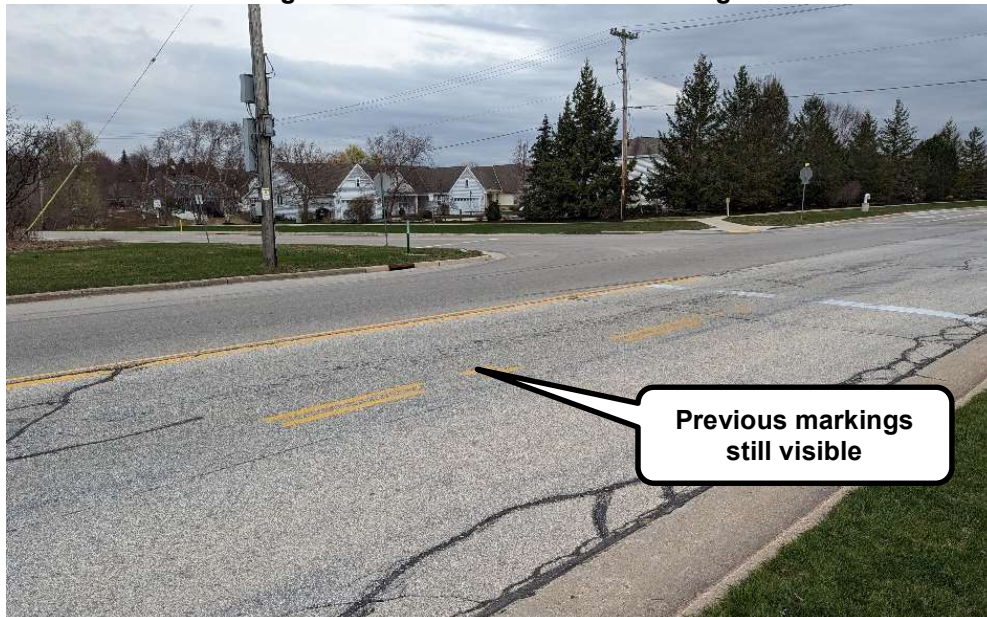
Figure 4: Previous Pavement Markings
