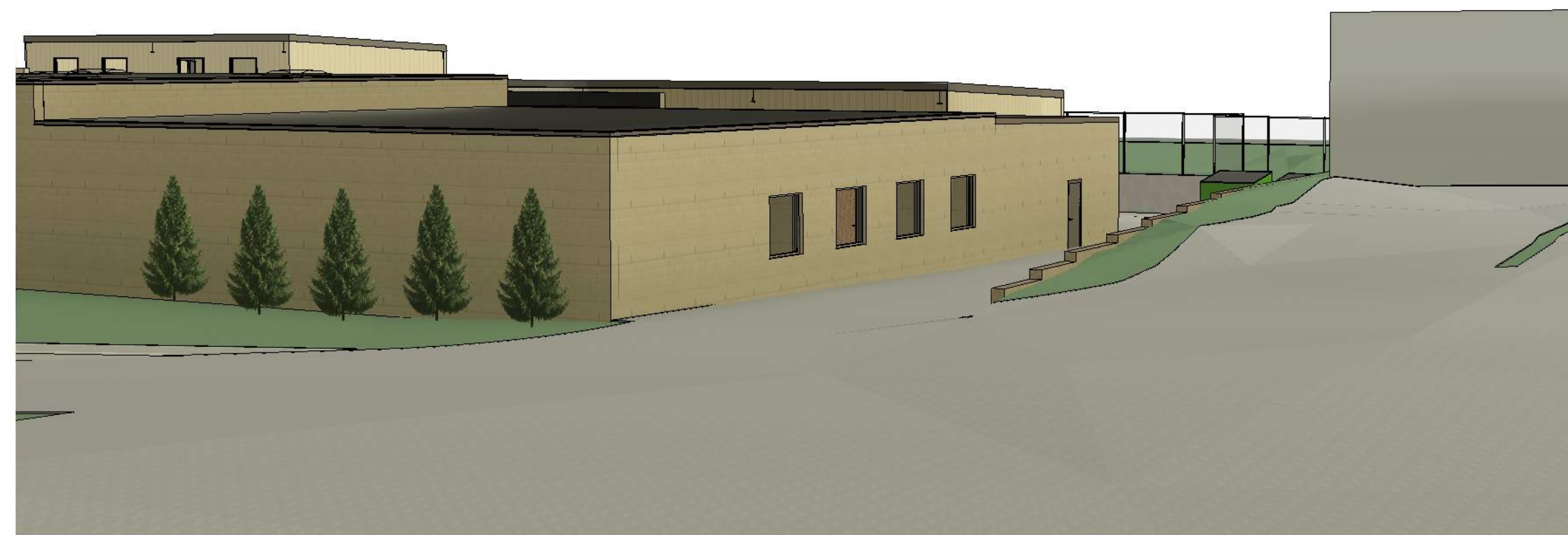
PARKING LOT VIEW
