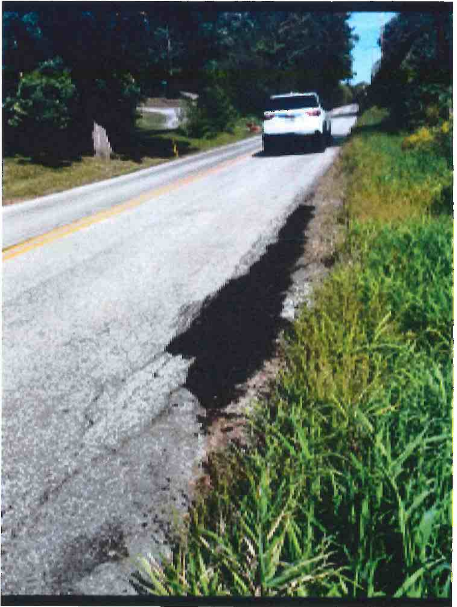
Hole Patched Picture Taken 9-13
