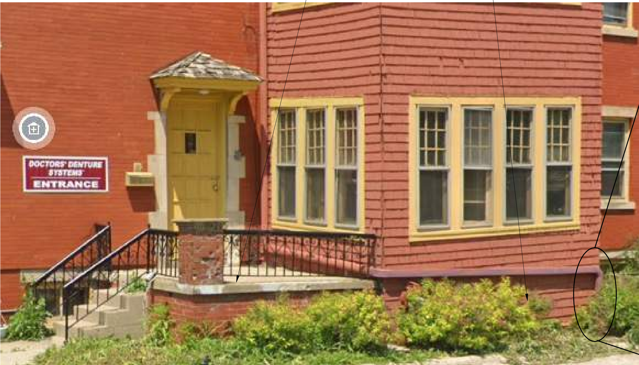
EXISTING SOUTH PORCH VIEW - WORK AREA
