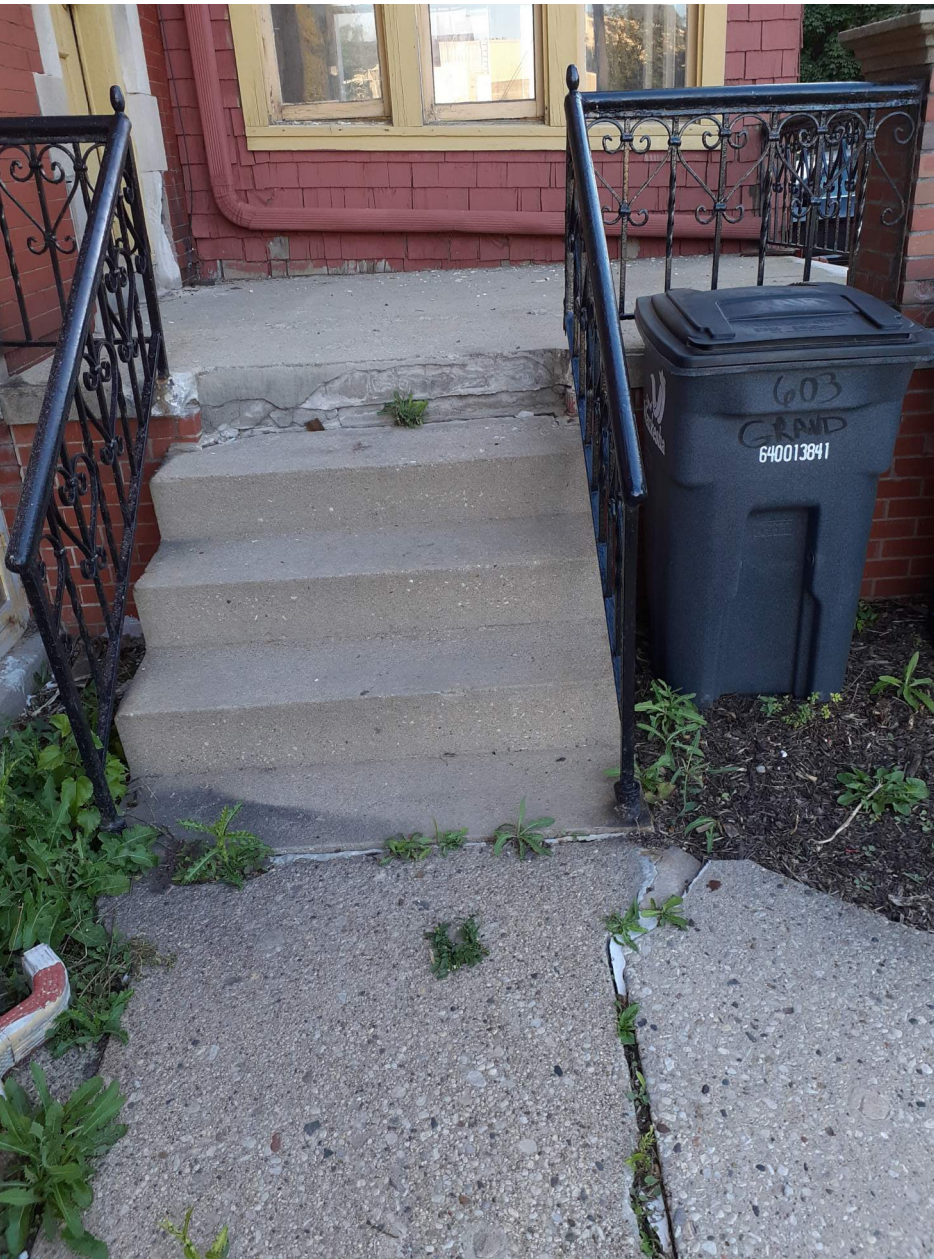
EXISTING PORCH STAIR & LANDING
