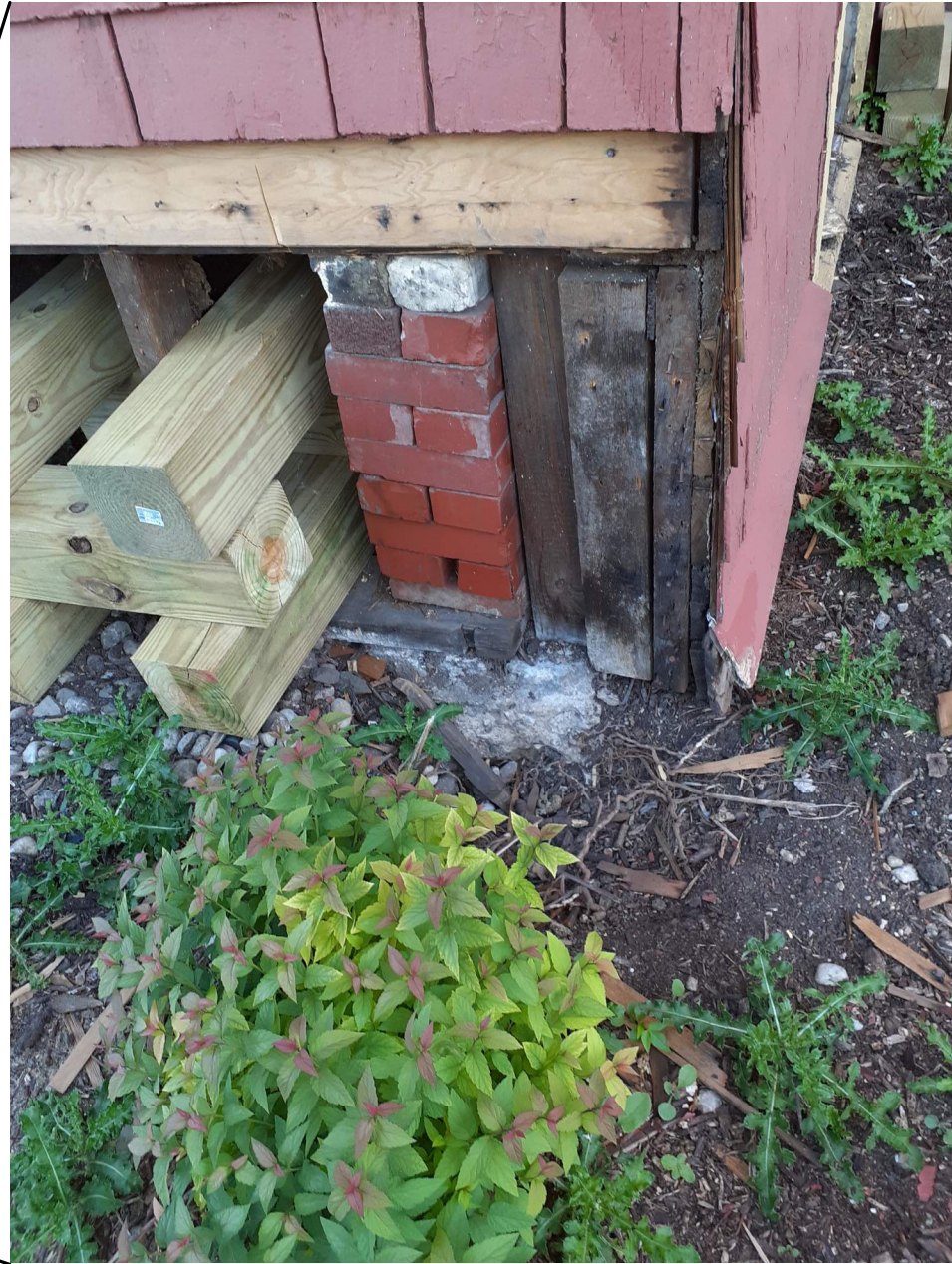
EXISTING SINKING FOUNDATION
