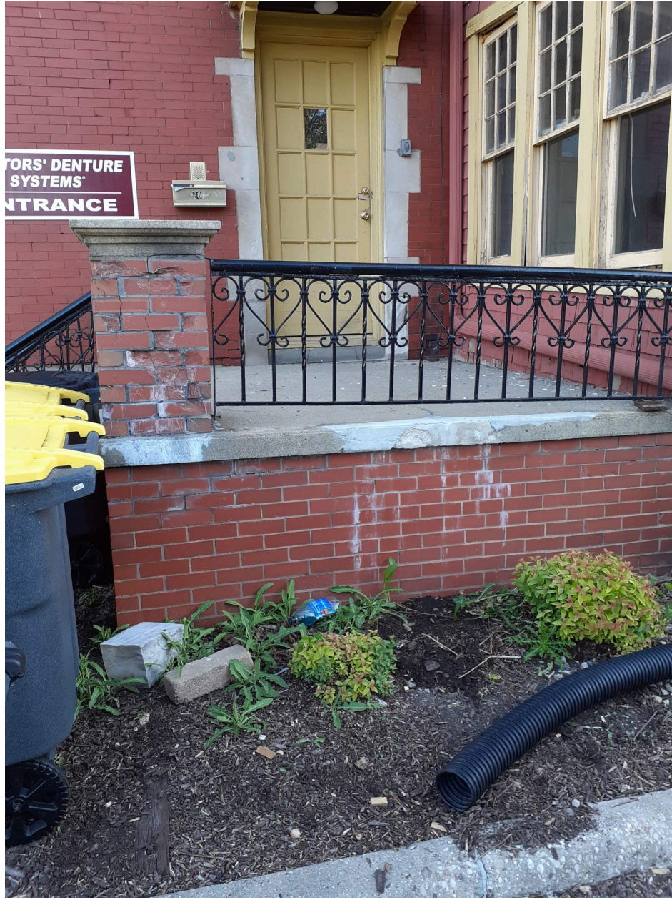
EXISTING PORCH RAIL / CORNER BRICK POST
