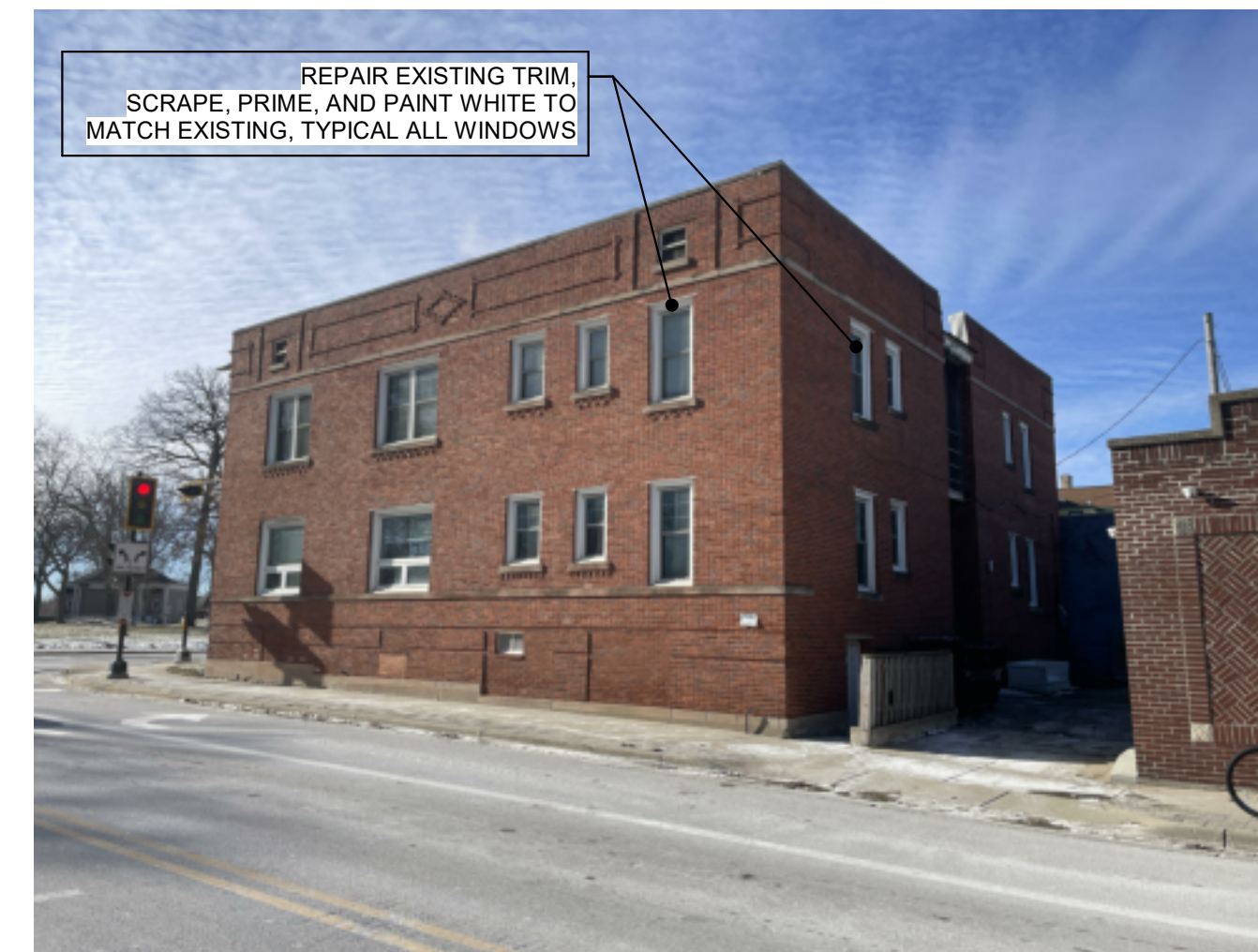
PHOTO 3 EXTERIOR NORTHEAST CORNER
