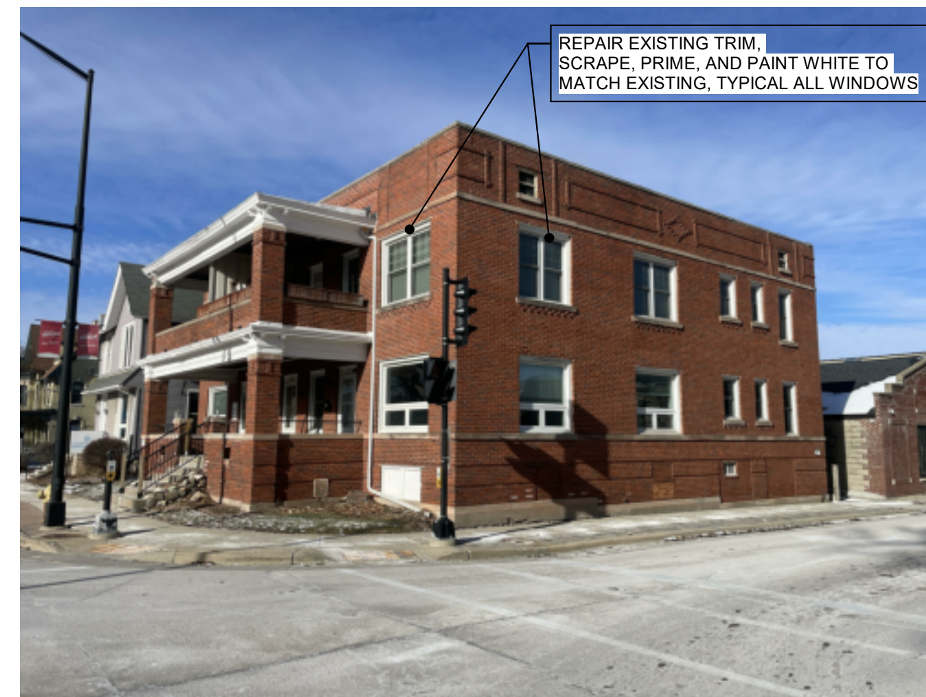
PHOTO 2 EXTERIOR SOUTHEAST CORNER
