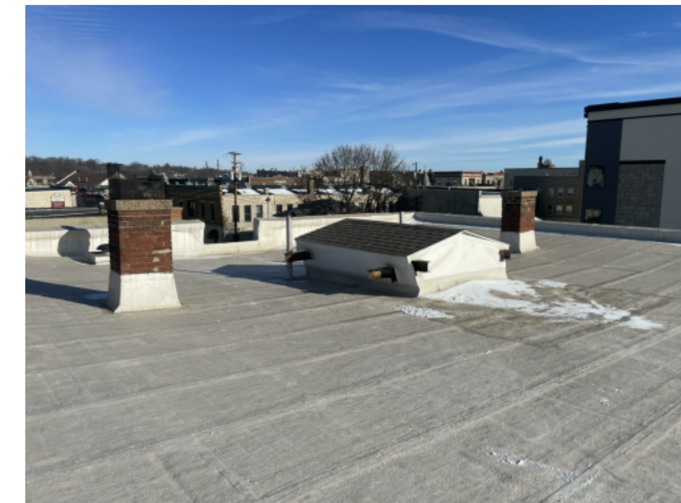
PHOTO 4 ROOF LOOKING NORTHEAST
