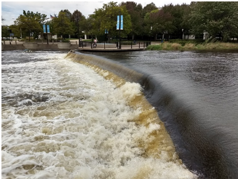
Saratoga Mill Dam 0063010031807.jpg Overflow Spillway from Left Abutment
