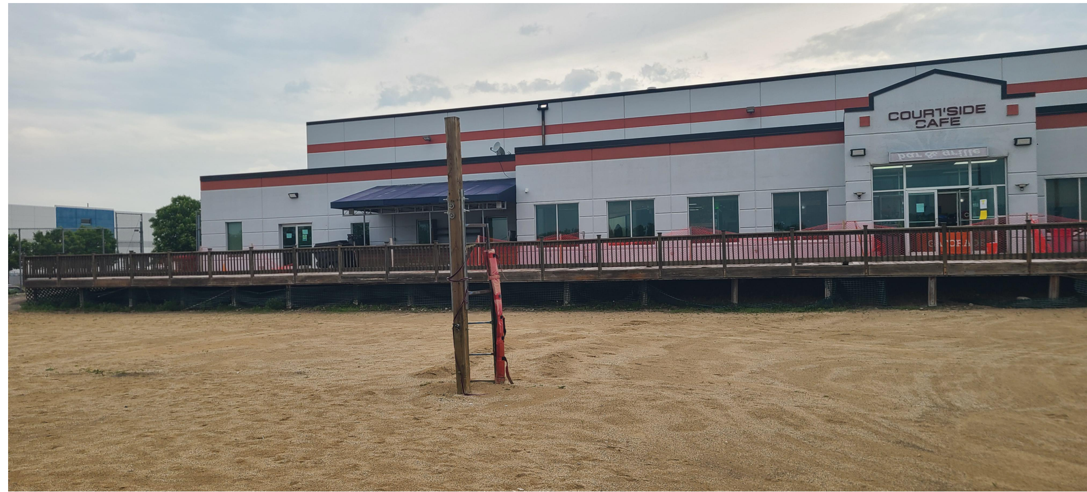
EXISTING DECK SOUTH ELEVATION
