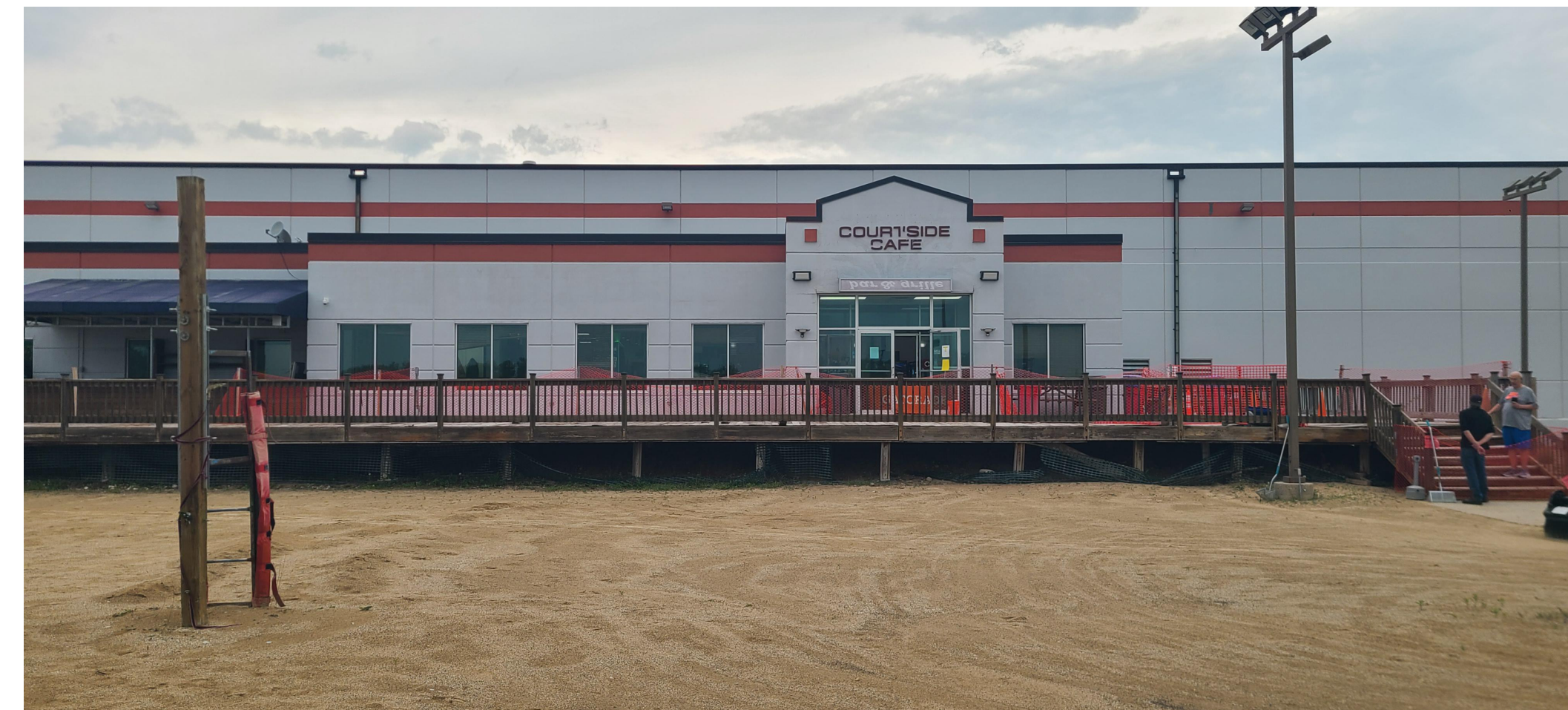
EXISTING DECK SOUTH ELEVATION
