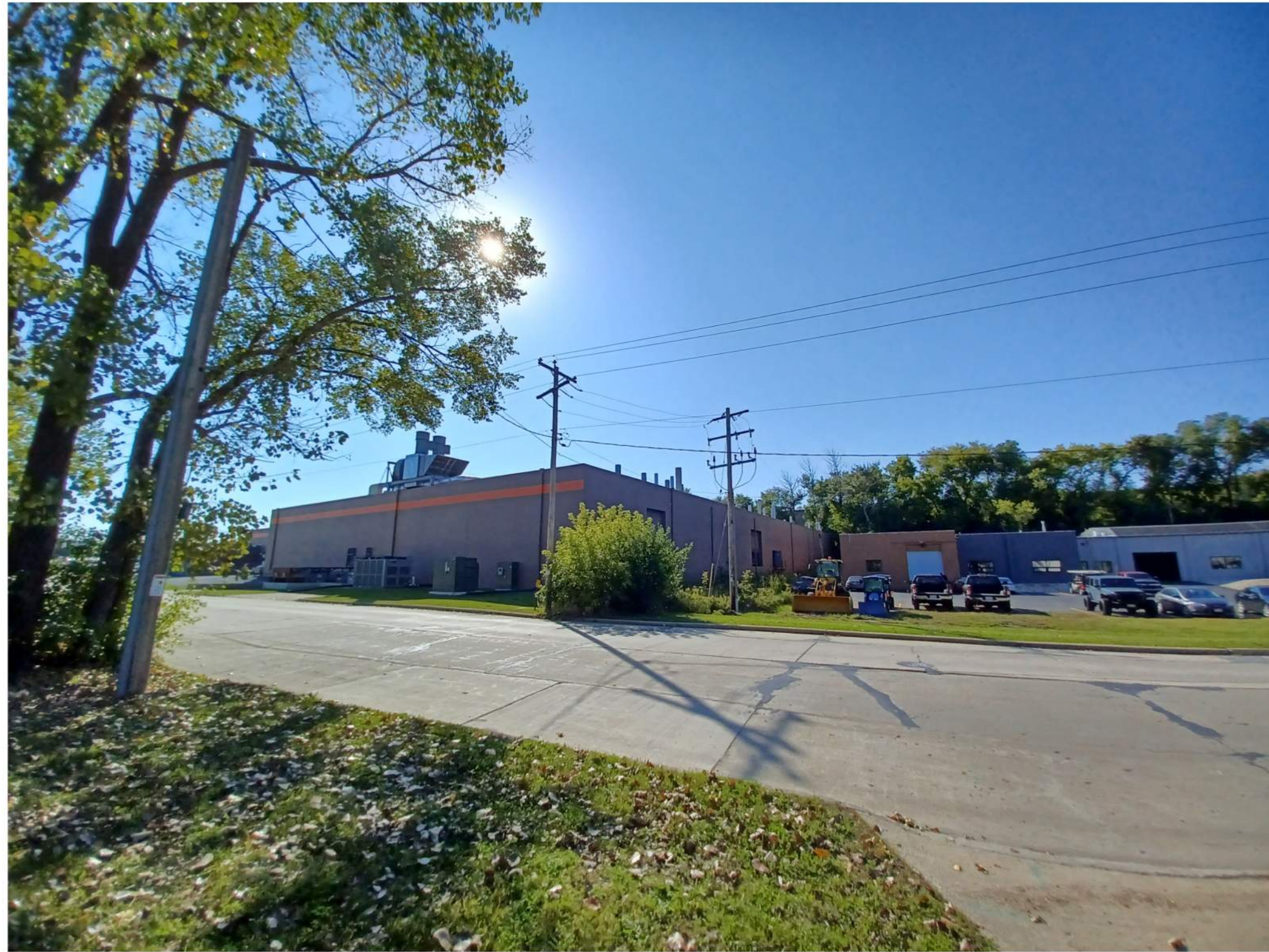
EXISTING SITE CONDITIONS FROM NORTHWEST CORNER
