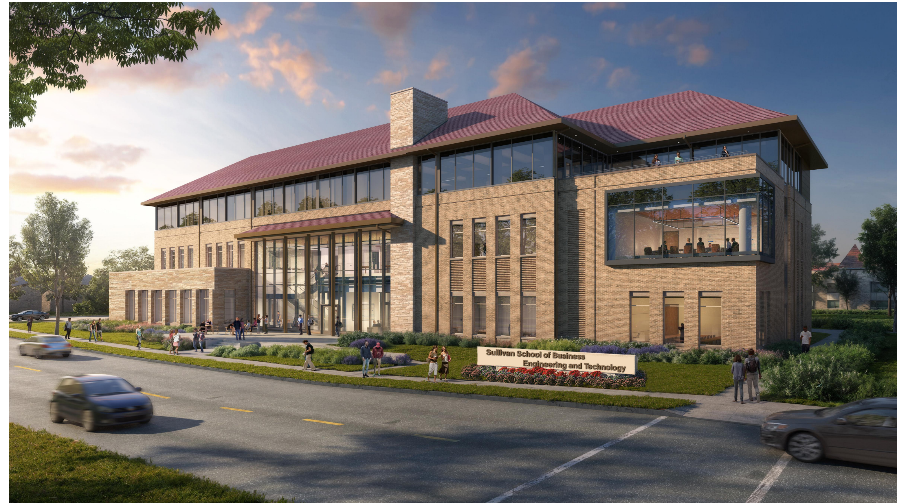
VIEW FROM BARSTOW STREET
