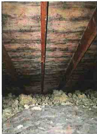
Possible Microbial Growth in Attic
