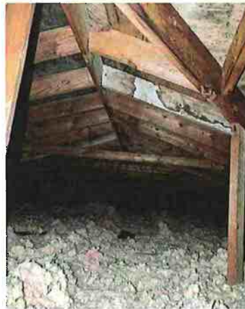
Possible Microbial Growth in Attic
