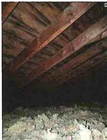
Possible Microbial Growth in Attic
