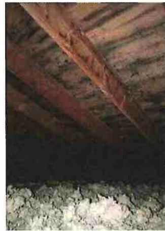
Possible Microbial Growth in Attic
